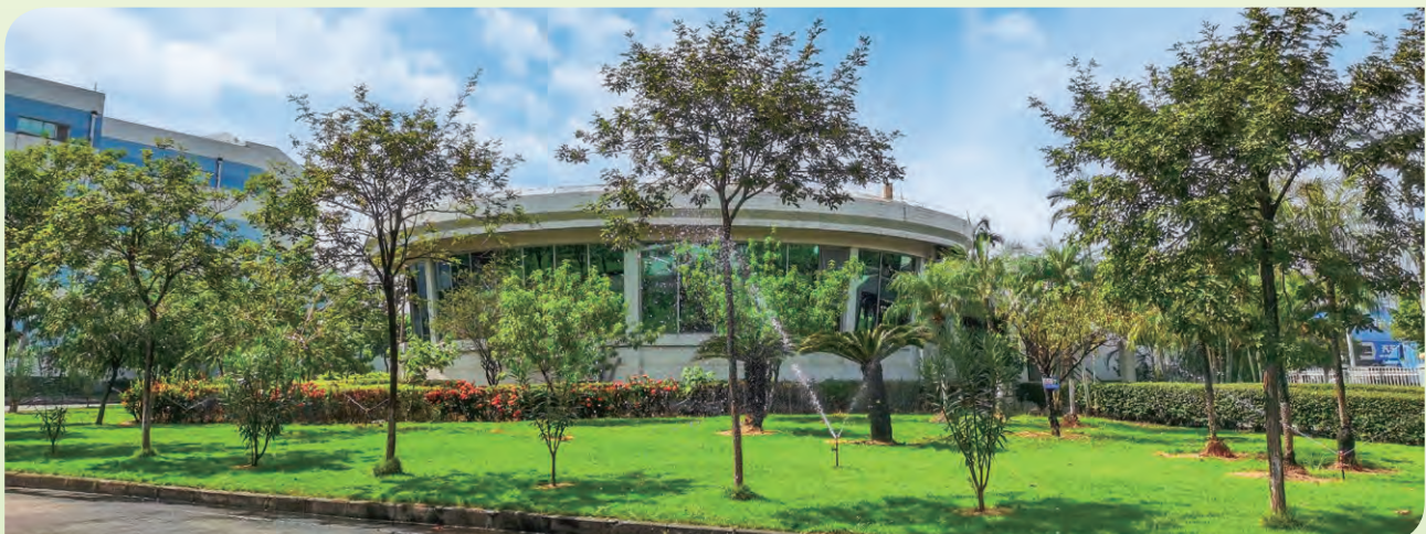
Rainwater Harvesting System at VTech Factory
