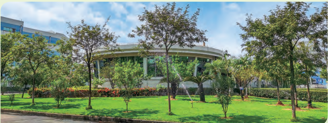
Rainwater Harvesting System at VTech Factory
