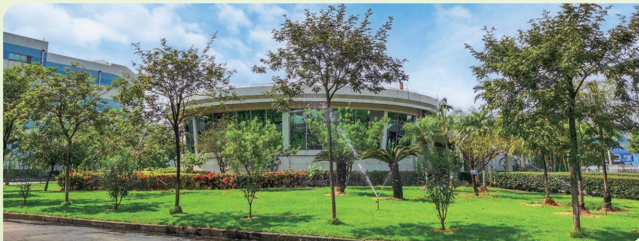
Rainwater Harvesting System at VTech Factory
